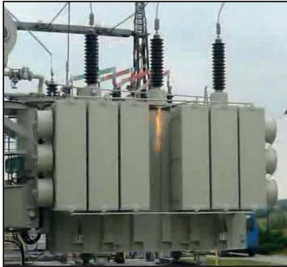
**Figure 2: Sparks on tank during inrush current, transformer 40 MVA, 110 kV**
