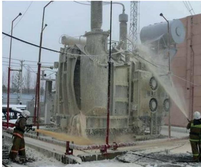
**Figure 4 – Transformer in Western Siberia Substation after explosion**
